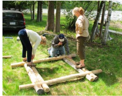
We laid it out, notched the posts and put it together like Lincoln logs. Added a wire mesh base to hold the nesting materials
