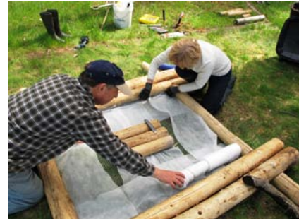
Laid a filter cloth across the bottom to retain soil for plants. Added the nesting & native plant material on top.
