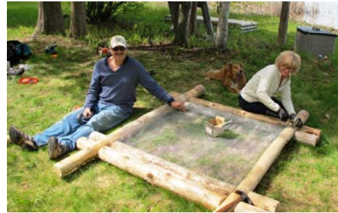
We laid it out, notched the posts and put it together like Lincoln logs. Added a wire mesh base to hold the nesting materials
