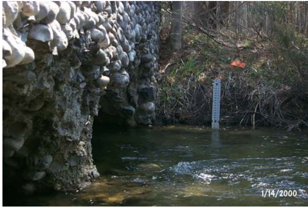
Platte River, Stone Bridge
